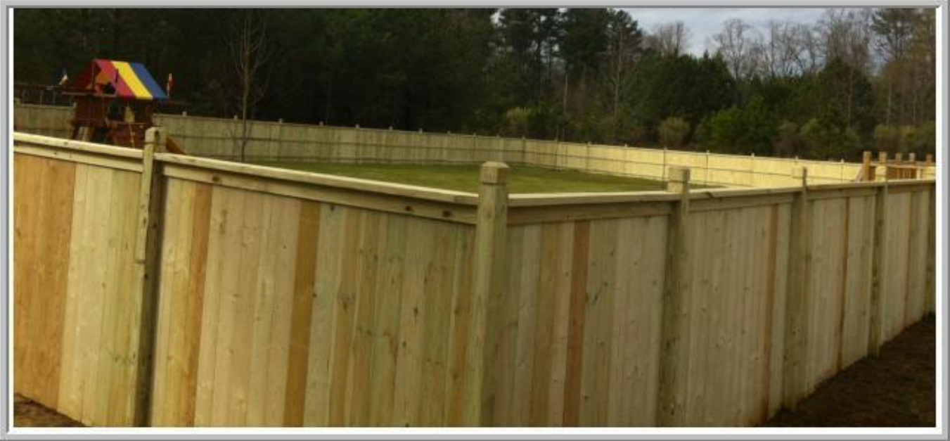
Cap Top with dado posts (Includes a horizontal 2x4 along the top of fence panels) (YES - PREFERRED)
